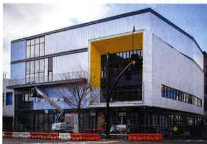
The Nashua Center for the Arts under construction
